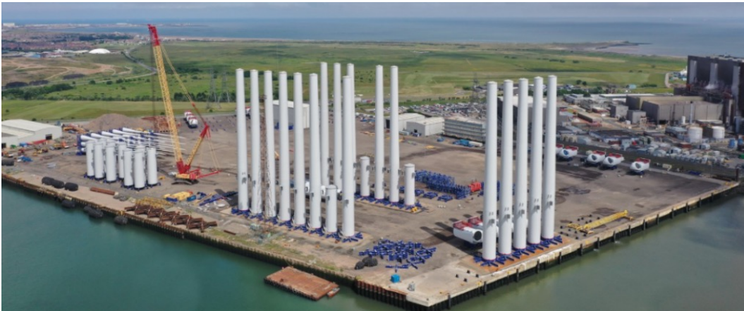
FIGURE 6: FIXED BOTTOM PORT, SOURCE: ABLE, UK
