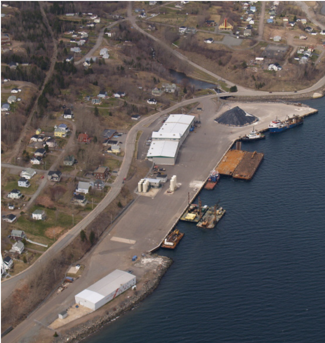
FIGURE 2: MULGRAVE MARINE TERMINAL, SOURCE STRAIT SUPERPORT CORPORATION
